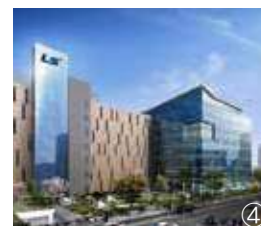
GYG Elevator installation site ( Domestic )
