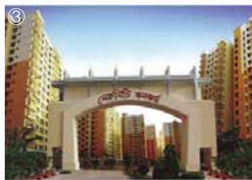
GYG Elevator installation site (overseas)
